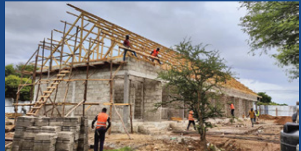
Married couple Hostel Construction on progress.
