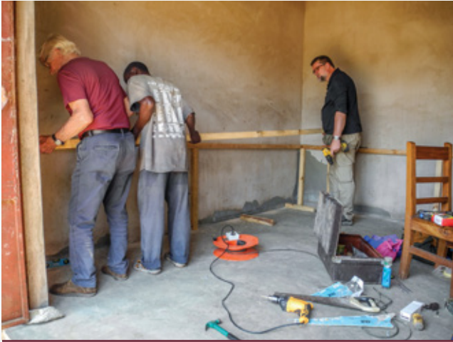
A team Constructing the shelves
