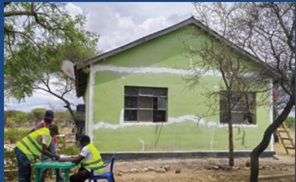
Domitories revonavation on progress
