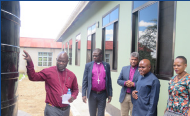
Bishop Dr. George Okoth, Archbishop of Sydney Kanishka Raffel and Bishop Musa yamo of Rorya Diocese inspecting water tank in new builded classroom at BBC.
